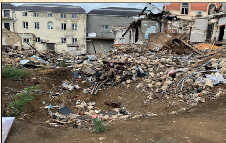
Destruction of Residential Complex in Ganja City
