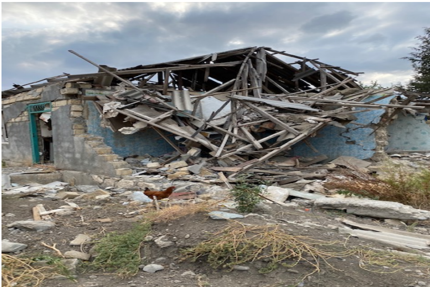
Damaged House in Terter City
